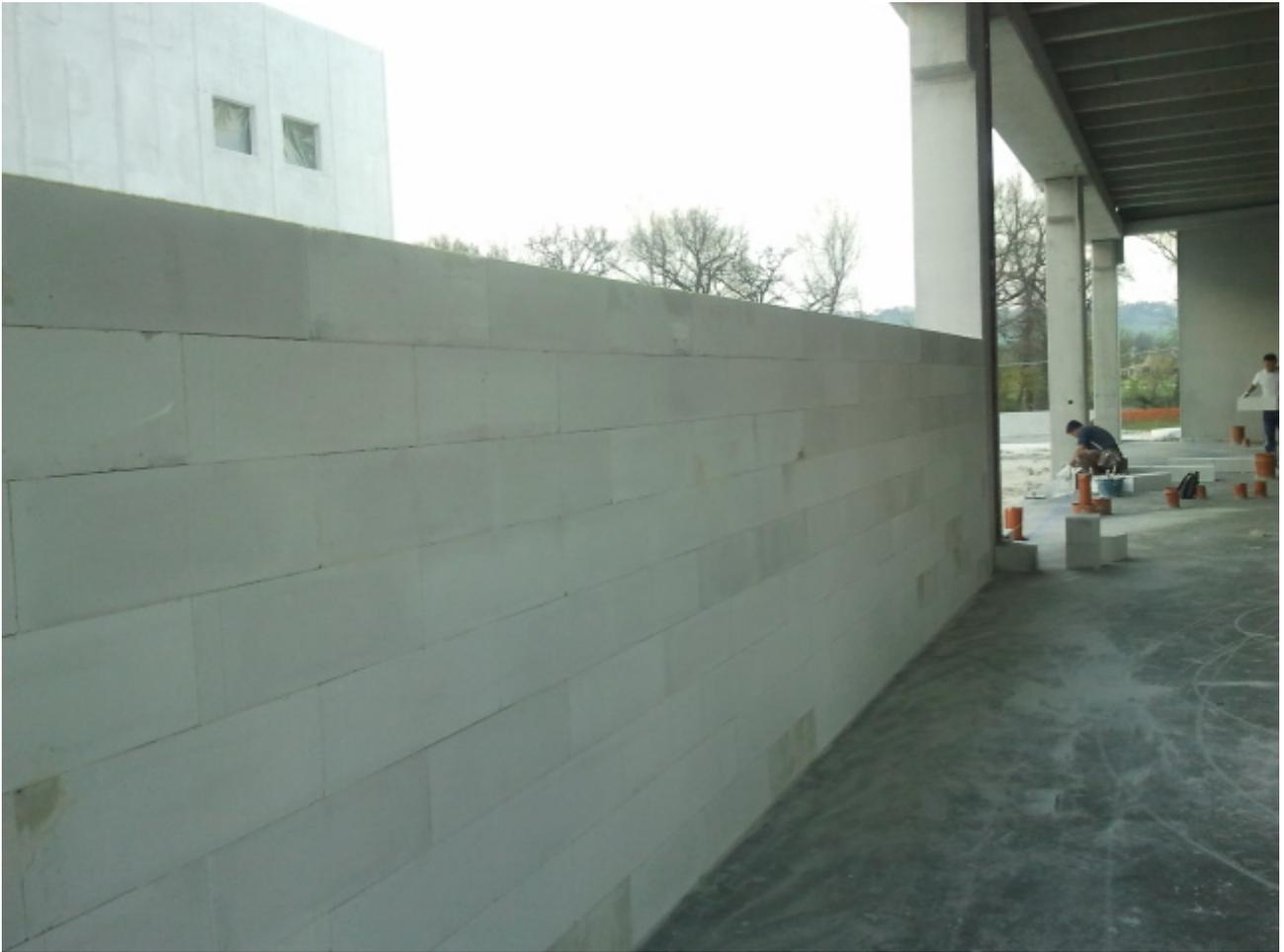
VISTA ESTERNA DELLA STRUTTURA IN ACCIAIO PER CORPO MC DONALD E TAMPONATA CON BLOCCHI DA CM.30 YTONG CHE VERRANNO SUCCESSIVAMENTE RASATI E RIVESTITE CON LASTRE IN FIBROCEMENTO PER ESTERNO.
